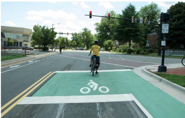
Bicyclist waiting at a signal in a bicycle box with optional green colored pavement
