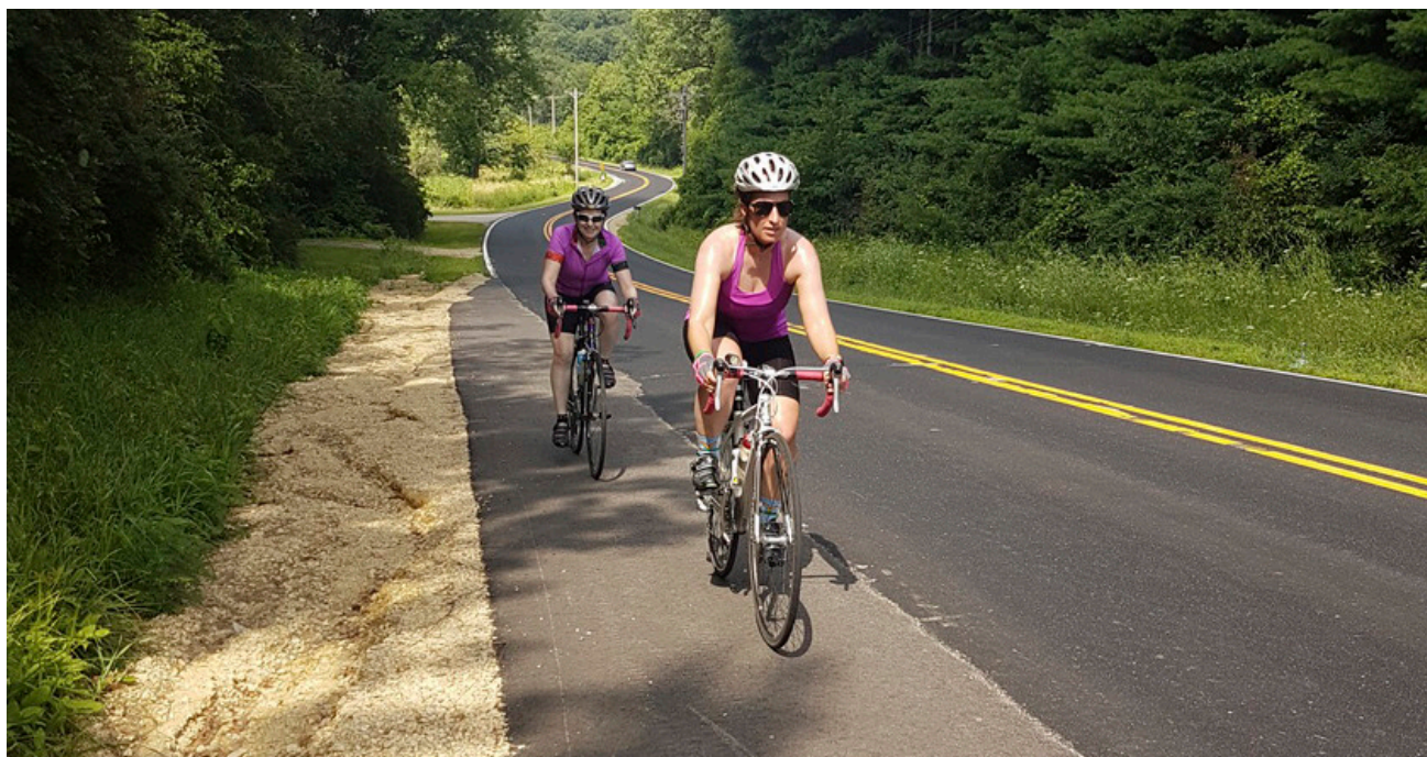
Shoulder widening along an uphill grade
