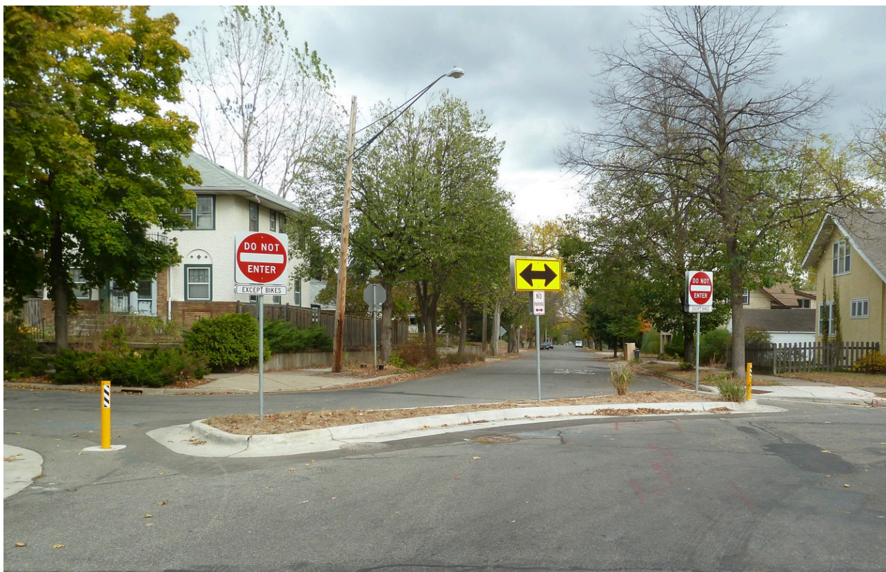
Traffic diverter at 11th Avenue S., Minneapolis, MN
