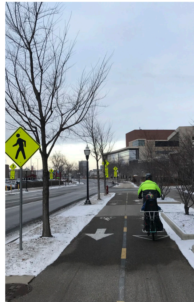
A separated bicycle lane in Minneapolis
