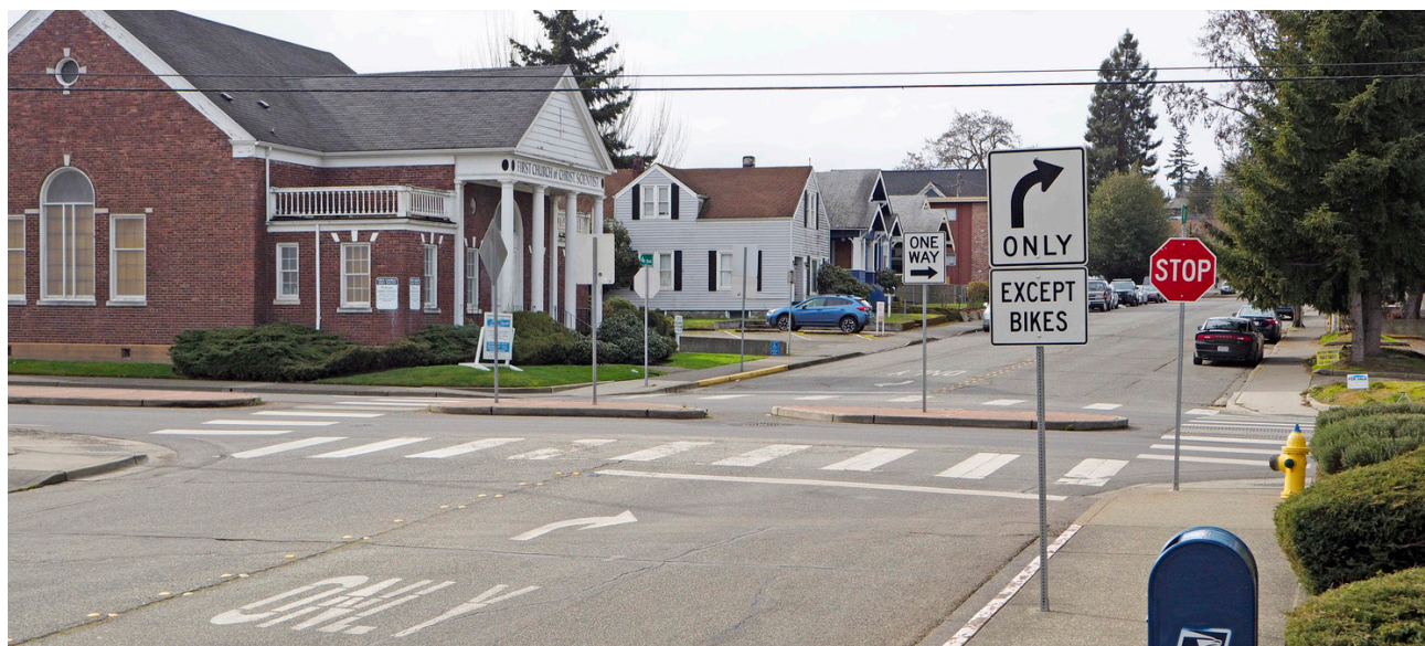
Traffic diverter with an opening for bicycles
