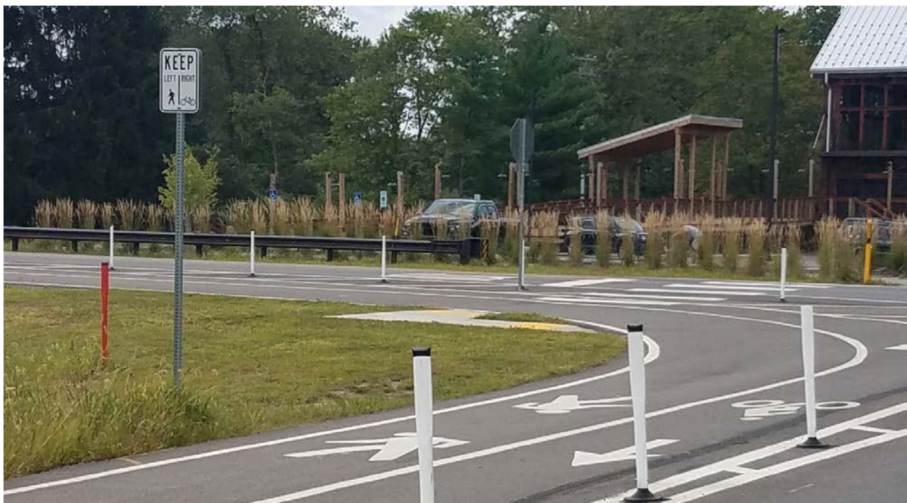
A temporary on-street shared use path
