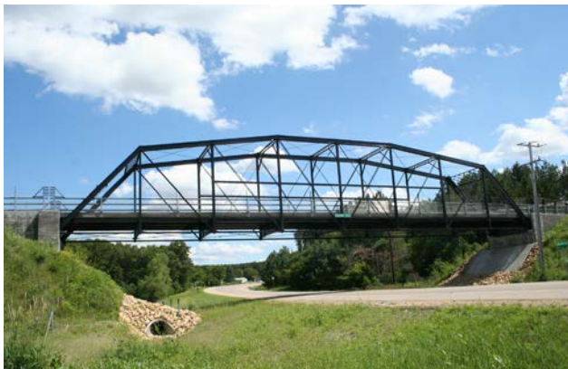
Gateway Trail Bridge, Washington County, MN; Source: MnDOT
