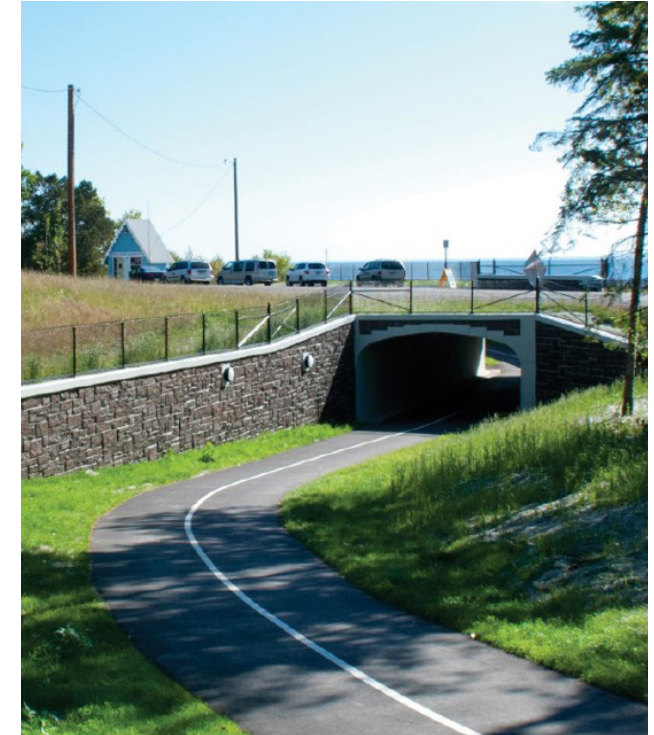
Lakewalk Trail tunnel under TH 61, Duluth, MN
