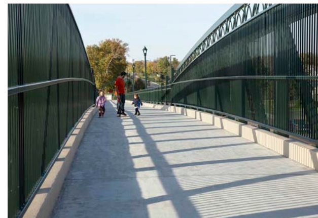
Bridge overpass at TH 23 & Saratoga Street, Marshall, MN
