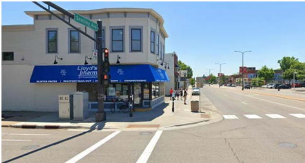
Curb retrofit on Snelling Avenue, Saint Paul, MN; Source: Google
