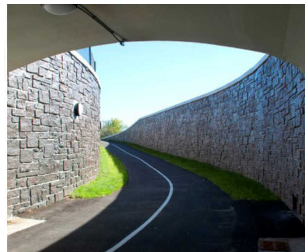
Lakewalk Trail tunnel under TH 61, Duluth, MN
