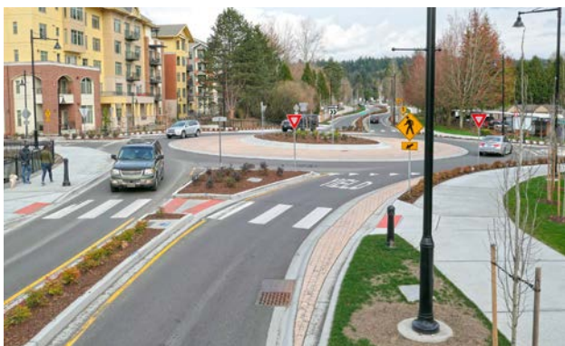
A pedestrian crossing at a roundabout
