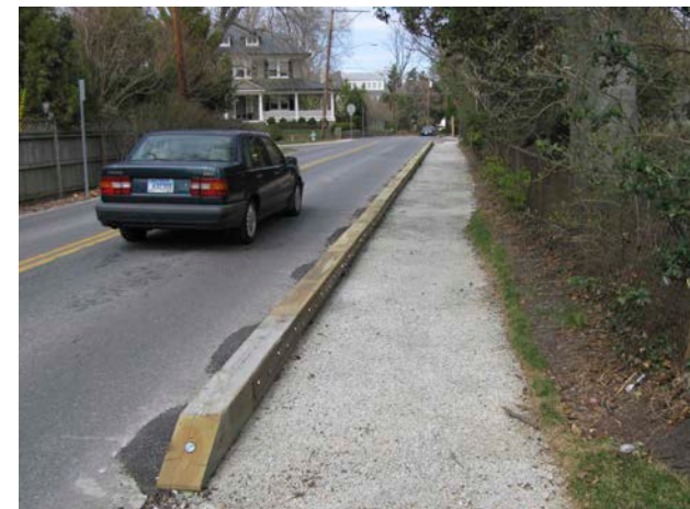
A temporary on-street shared use path
