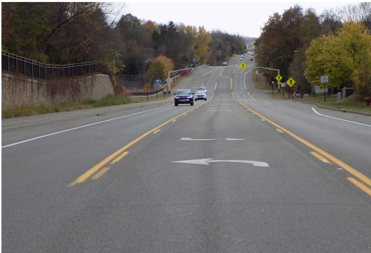
Road diet with RRFB on CR-101 S, Minnetonka, MN
