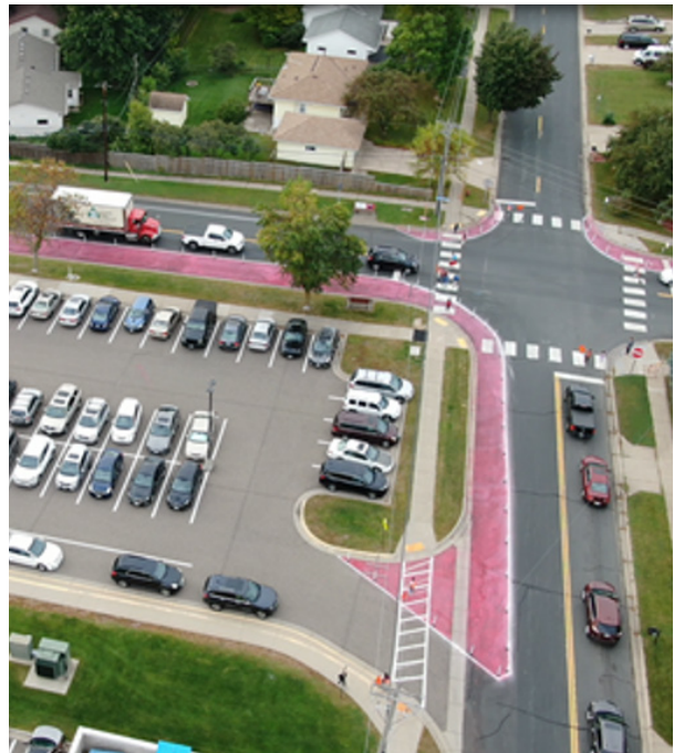
Image 4.12: Right-turn lane removal and curb extensions demonstration project
