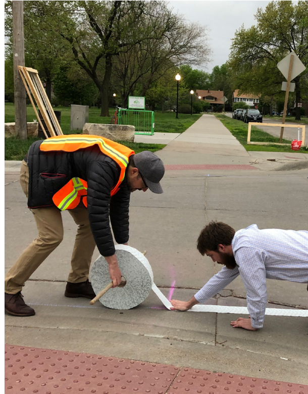
Image 7.01: Application of traffic tape
