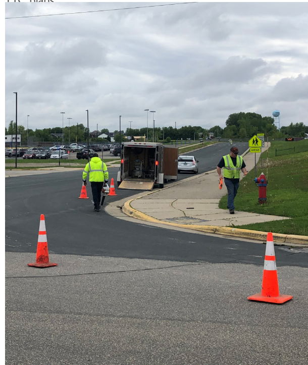
Image 5.05: Temporary traffic control during demonstration project installation
