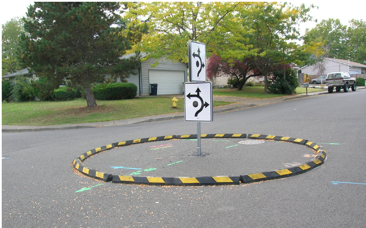
Image 4.11: Example of a mini traffic circle constructed with parking stops and signs
