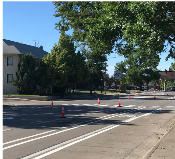
Image 4.13: Traffic lane conversion from 4 to 3 lanes with buffered bike lanes
