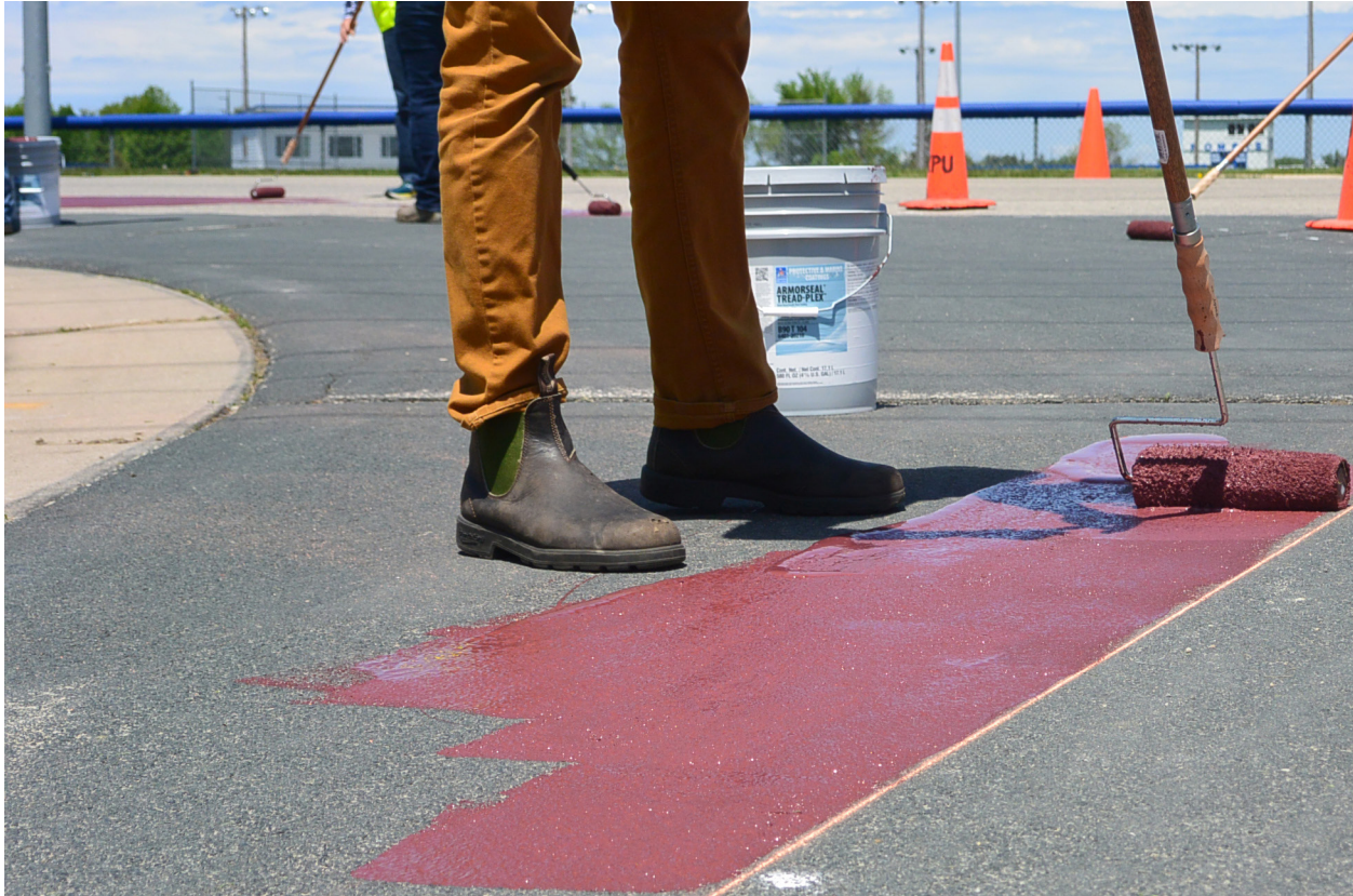
Image 3.02: Applying paint to street with roller and extension handle
