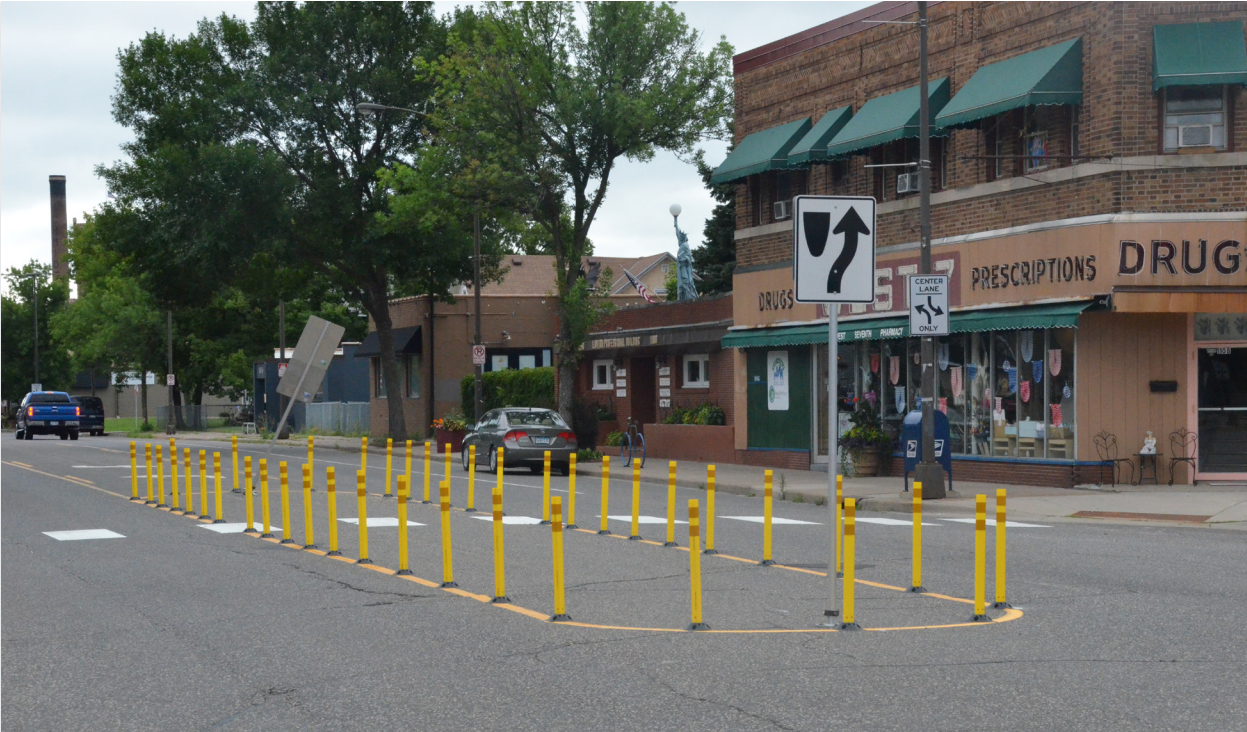
Image 4.07: Example of a median safety island (pedestrian refuge island)
