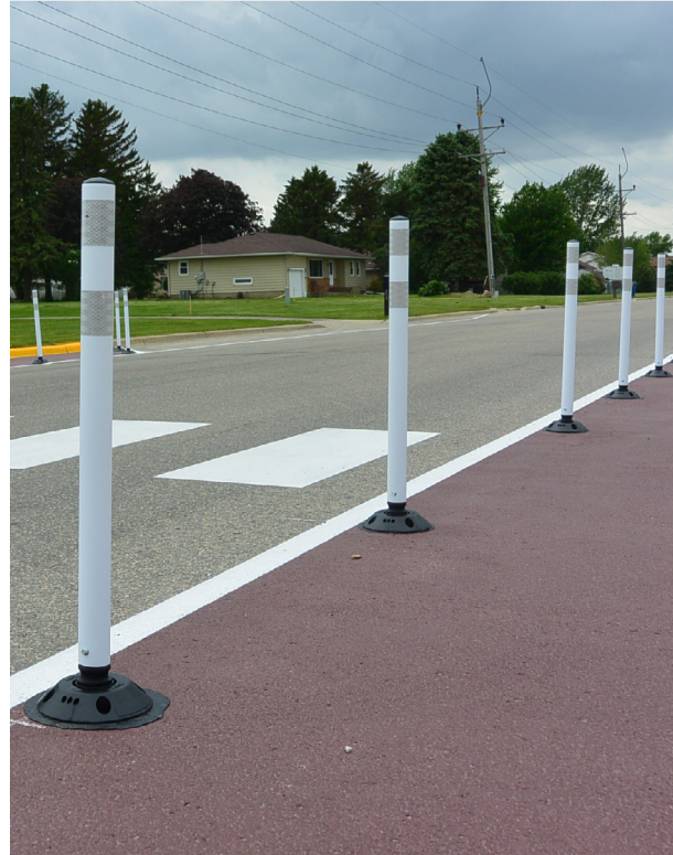
Image 7.02: Flex posts installed with butyl pods
