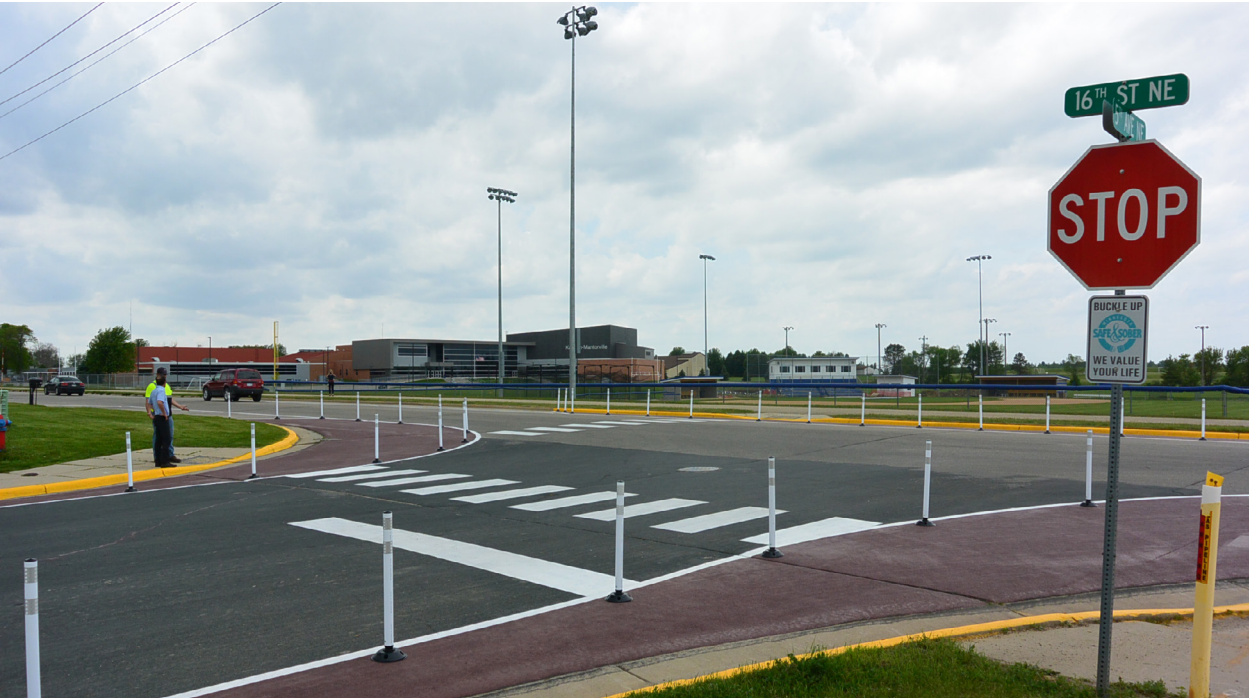
Image 4.03: Stop line installation
