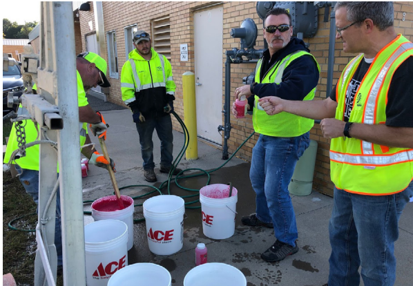
Image 3.01: A demonstration project installation team prepares paint
