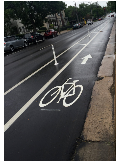
Image 4.10: Example of a separated bike lane
