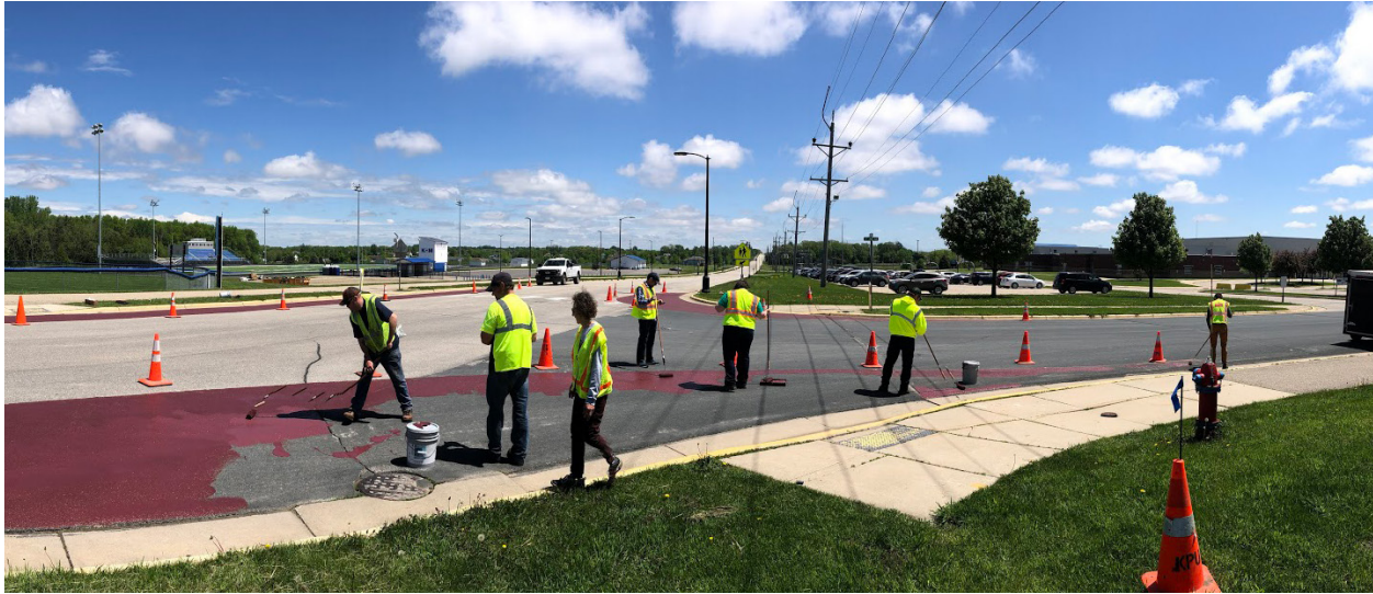
Image 6.03: Photograph from demonstration project installation - Kasson, MN
